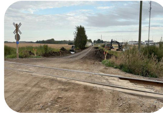
Rail Crossing Improvements
