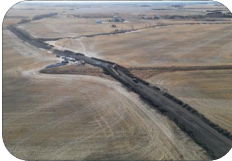
Villeneuve Drainage – Phase 4B
