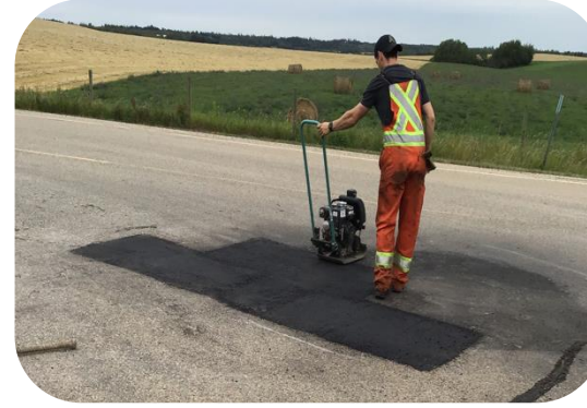
Paved Road Maintenance
