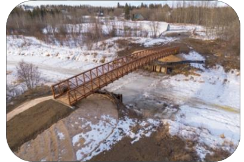
Casa Vista Pedestrian Bridge
