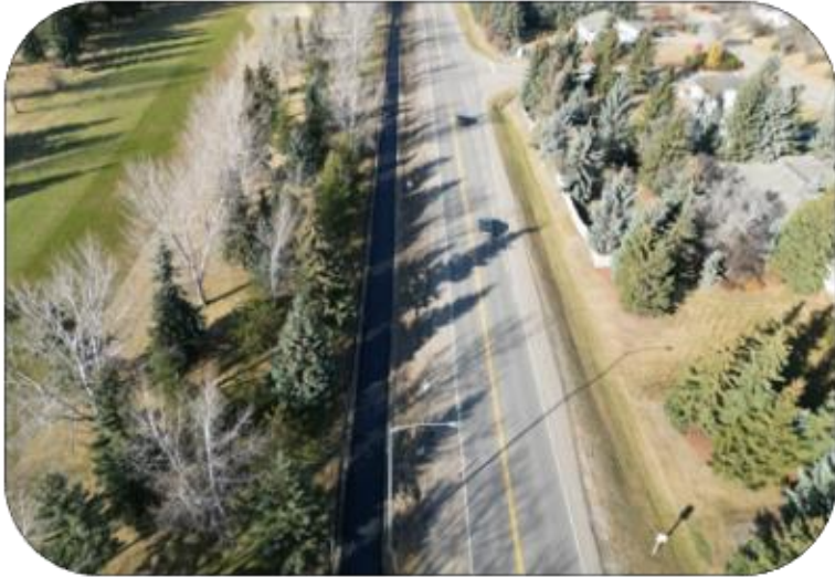
Starkey Rd Pedestrian Bridge and Pathway (2025/26)
