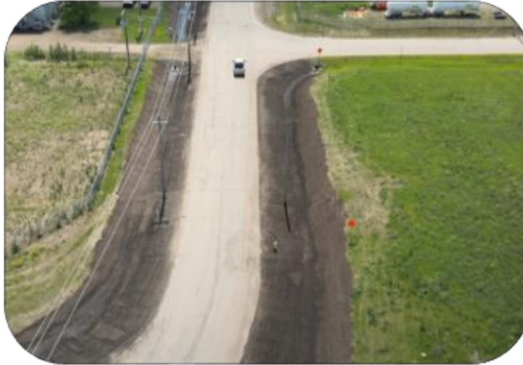
SIP Drainage Phase 3
